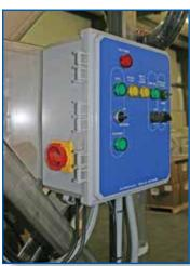
Master panel with automatic and manual pump control, hydraulic cleanout control, illuminated lights and lockout. Weather tight enclosure and waterproof switches.
